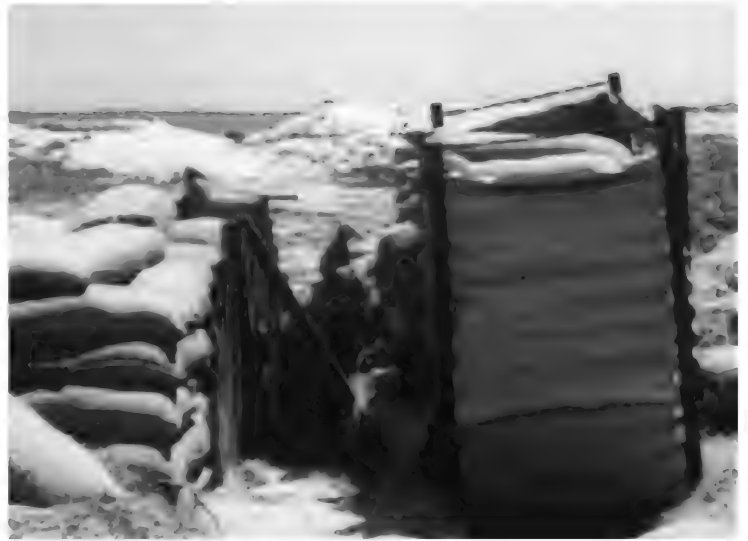
Left: Fig. 12.3, Andersons at 1800 ft after burst. Right: Fig. 12.4, Andersons protected by blast walls at 2760 ft.
